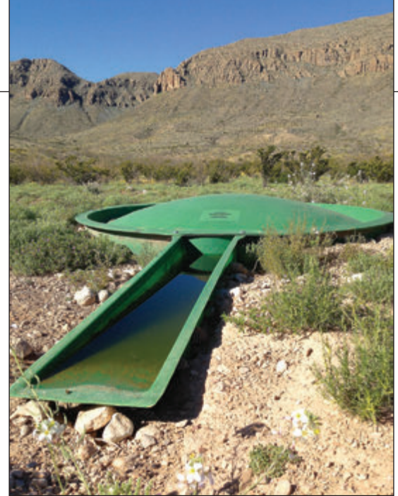
This Reservoir stores rainwater for the dry season.
